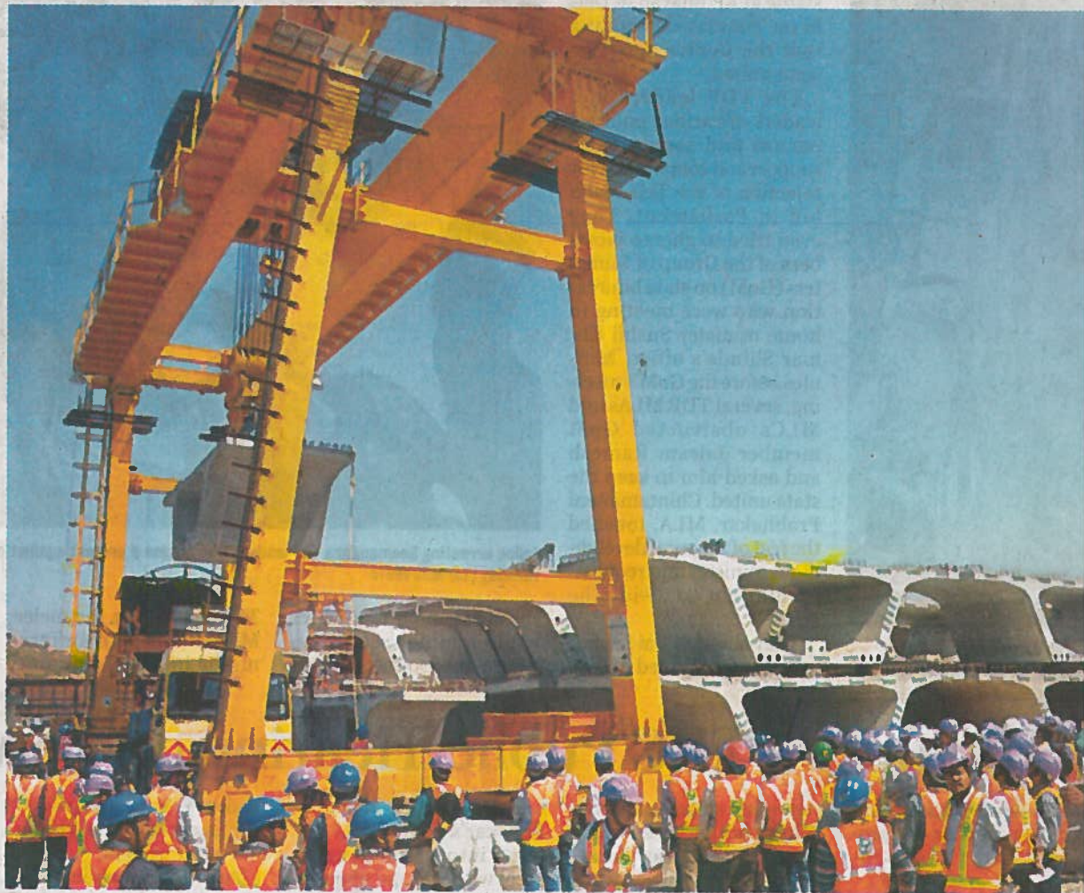
Viaduct segments for Hyderabad Metro Rail project being manufactured at Quthbullapur casting yard in Hyderabad on Tuesday | RVK RAO
