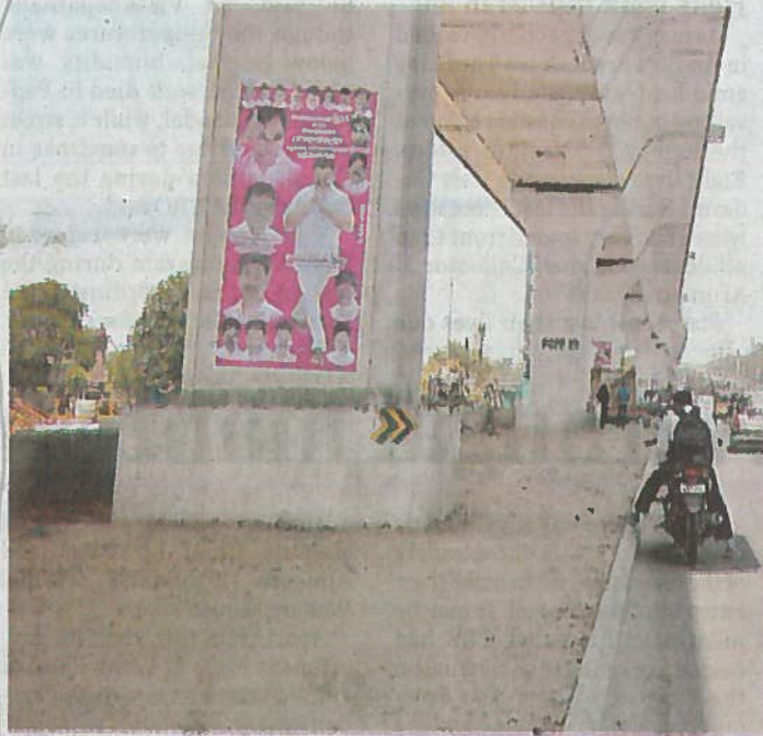
Posters on the pillars of Metro Rail tracks
