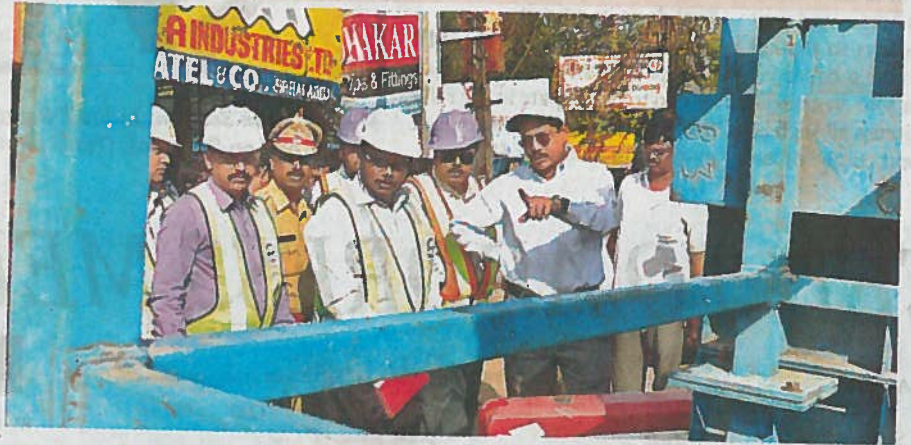
NVS Reddy, MD, HMR, inspecting Metro rail works at Bharat Nagar in Hyderabad on Saturday. (Hans photo)
