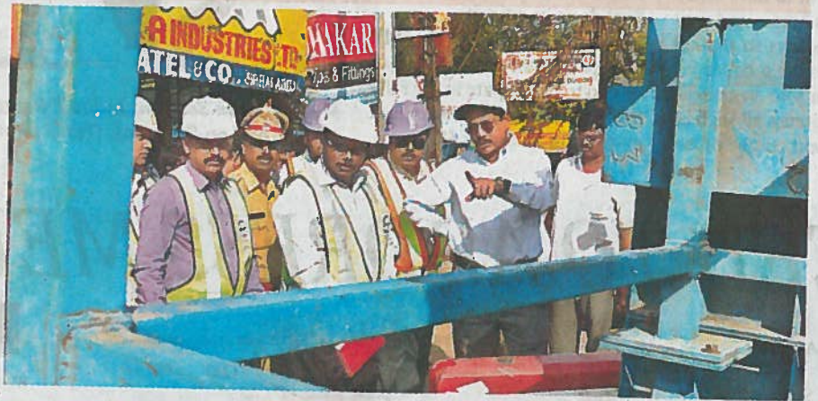
NVS Reddy, MD, HMR, inspecting Metro rail works at Bharat Nagar in Hyderabad on Saturday. (Hans photo)
