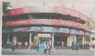
Garden restaurant demolition by May end
