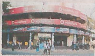
Garden restaurant demolition by May end
